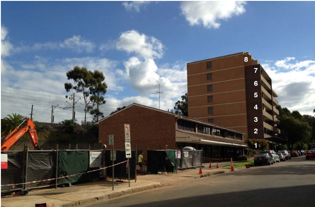
11 Hunter Street, Parramatta - construction to left of photo. 1 Hunter Street is in the background.
